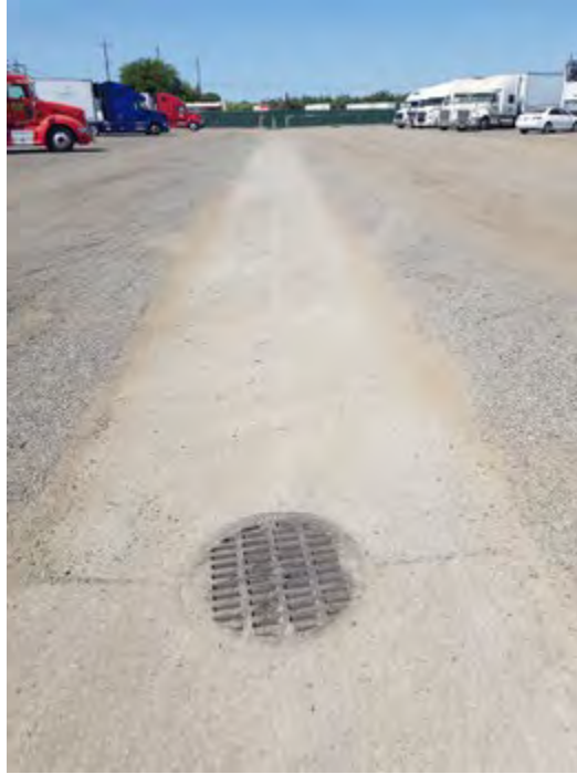
Figure 2.2-13 Sangha Trucking Yard Storm Drain
