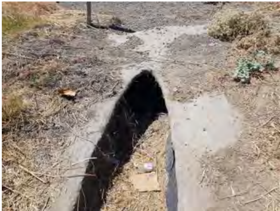
Figure 2.2-4 Sandhu Brothers Yard Culvert
